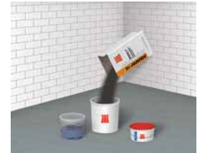
4 Filling out the waterproofing membrane at the pre-determined mix ratio
