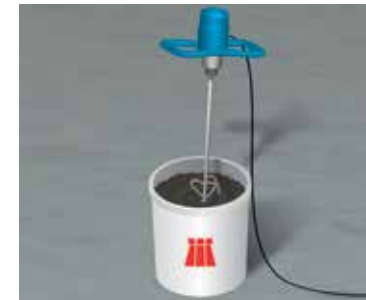
5 Mixing the waterproofing membrane
