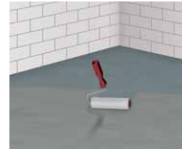
3 Priming the substrate, e.g. with ASO®-Unigrund
