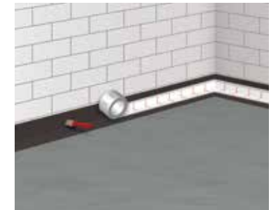
6 Bonding the ASO®-Joint-Tape into the first coat of the waterproofing membrane
