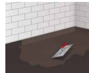
9 Application of the second coat of waterproofing membrane
