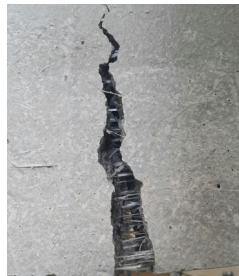
LEKSO 410 enhances the post-peak load carrying capacity of concrete by bridging the cracks (See ASTM C1018 toughness indices) (4 kg/m 3 fibre dosage)
