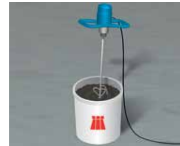
5 Mixing the waterproofing membrane
