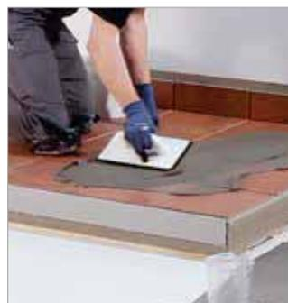
Grouting the tiles with ASO®Flexfuge.
