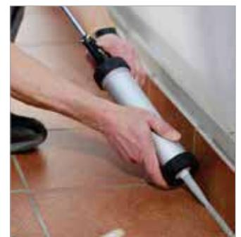
Elastic jointing with a suitable closed cell backing strip and sealing with ESCOSIL-2000.
