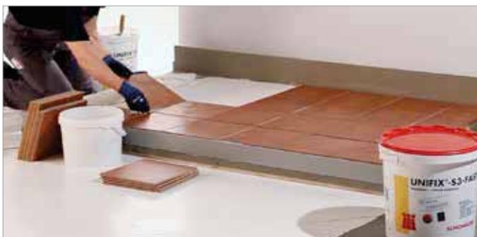
Sliding the tiles into the adhesive bed using the floating-buttering method.
