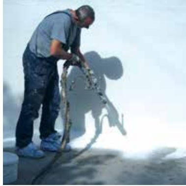
Spray application of a swimming pool
