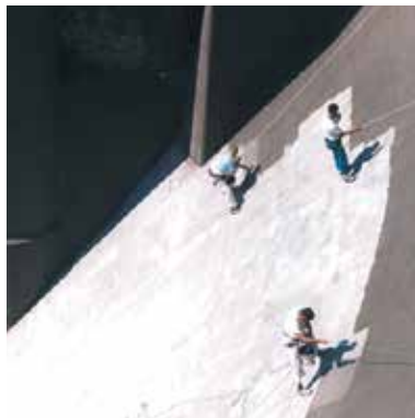
Brush application on a dam
