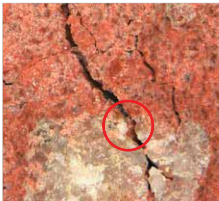
Crack formation in the concrete surface
