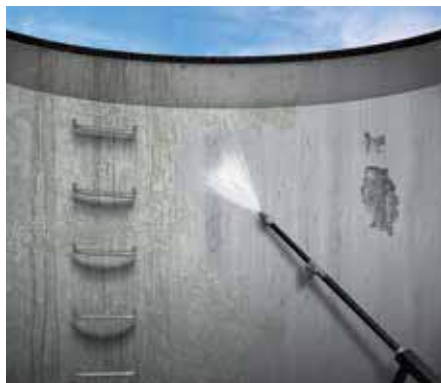
1 Cleaning prior to renovation
