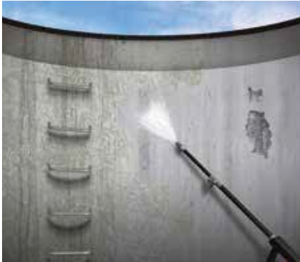
1 Cleaning prior to renovation
