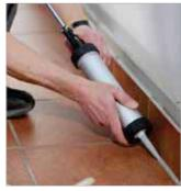
Elastic jointing with a suitable closed cell backing strip and sealing with ESCOSIL-2000.
