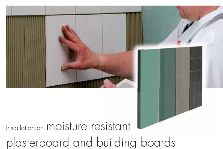
Moisture resistant plasterboard is only suitable as a substrate for exposure class AO, i.e. for moderately wet wall areas in rooms where splash contact and cleaning water is present, e.g. domestic bathrooms. The building board is to be protected against moisture damage with a bonded waterproof membrane.
