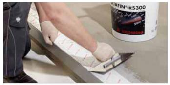
Incorporating the system's waterproof tape ASO®-Joint-Tape-2000-S into AQUAFIN®-RS300 on a balcony end profile.
