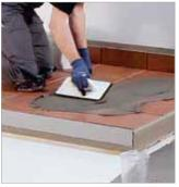
Grouting the tiles with ASO®-Flexfuge.
