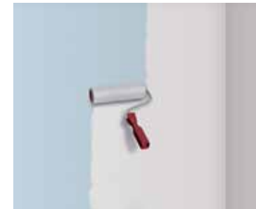
3 Priming the substrate, e.g. with ASO®-Unigrund
