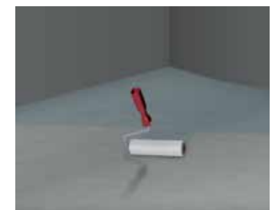
8 Priming the substrate, e.g. with ASO®-Unigrund
