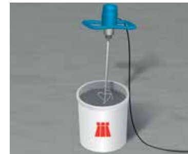
5 Mixing the smoothing compound
