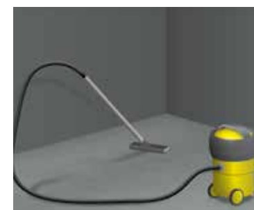
7 Cleaning the floor substrate
