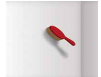
2 Cleaning the wall substrate
